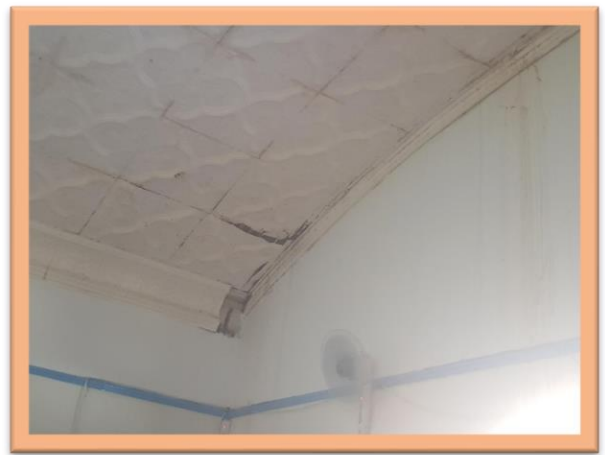
Condition of interior ceiling
