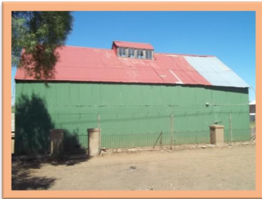
Main building – exterior view
