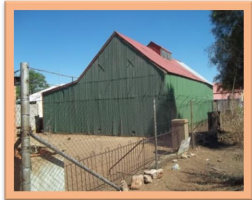
Main building – exterior view
