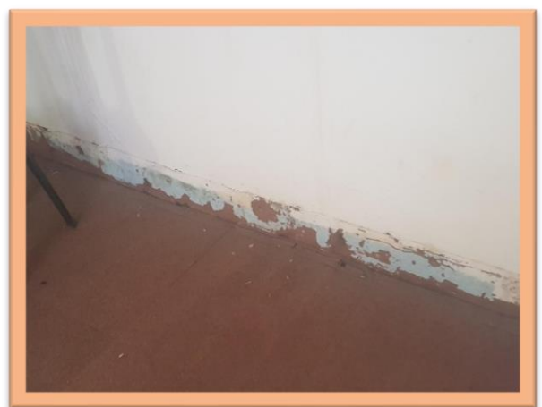
Interior flooring and skirting
