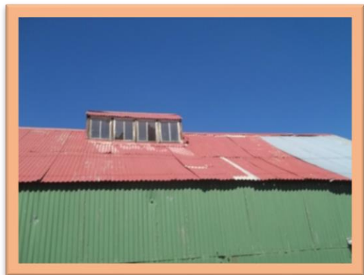
Main building - Roof
