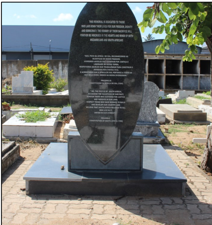
Fig. 1 This shield gives an idea/example of how a shield headstone can be erected. The bottom part would need to be 800mm wide should this model be chosen.
