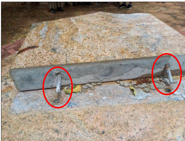
Fig. 2 Reinforcement Steel rods under the pillars
