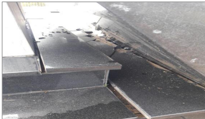
Fig.2 Base of the grave damaged by a falling granite plaque.
