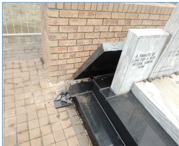
Fig.3 The granite plaque that fell from the memorial wall damaging the grave.
