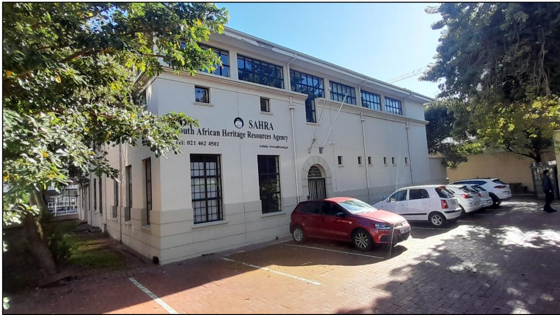
Figure 5: Photo of car park show access door for BH 2
